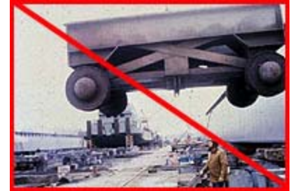
Improper practice: Worker exposed to overhead load.
