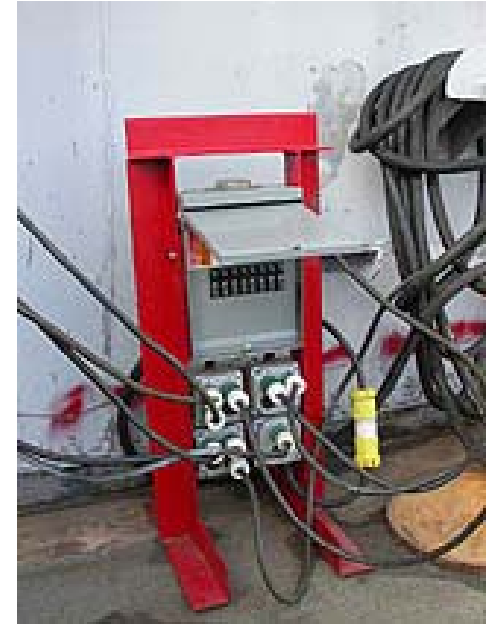
Circuit breakers used with temporary electrical power supplied to ship.
