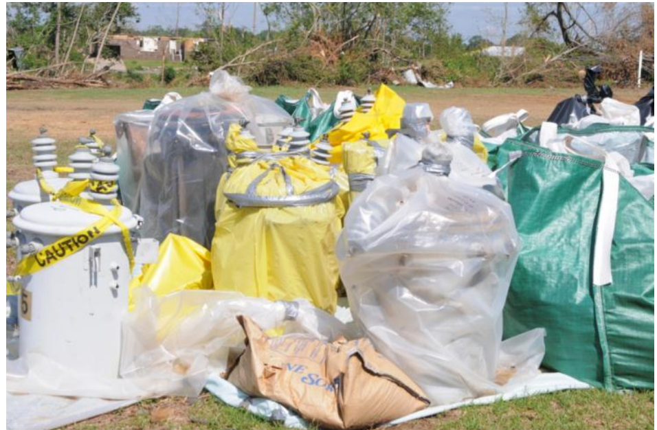
Transformers and other electrical equipment wrapped in bags to prevent oils from leaking
