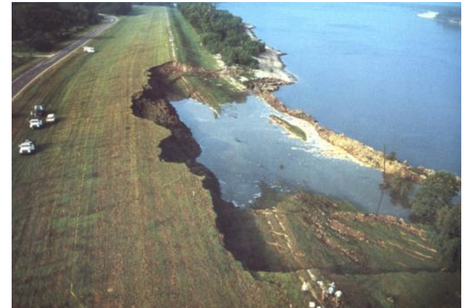
Picture of levee breach
