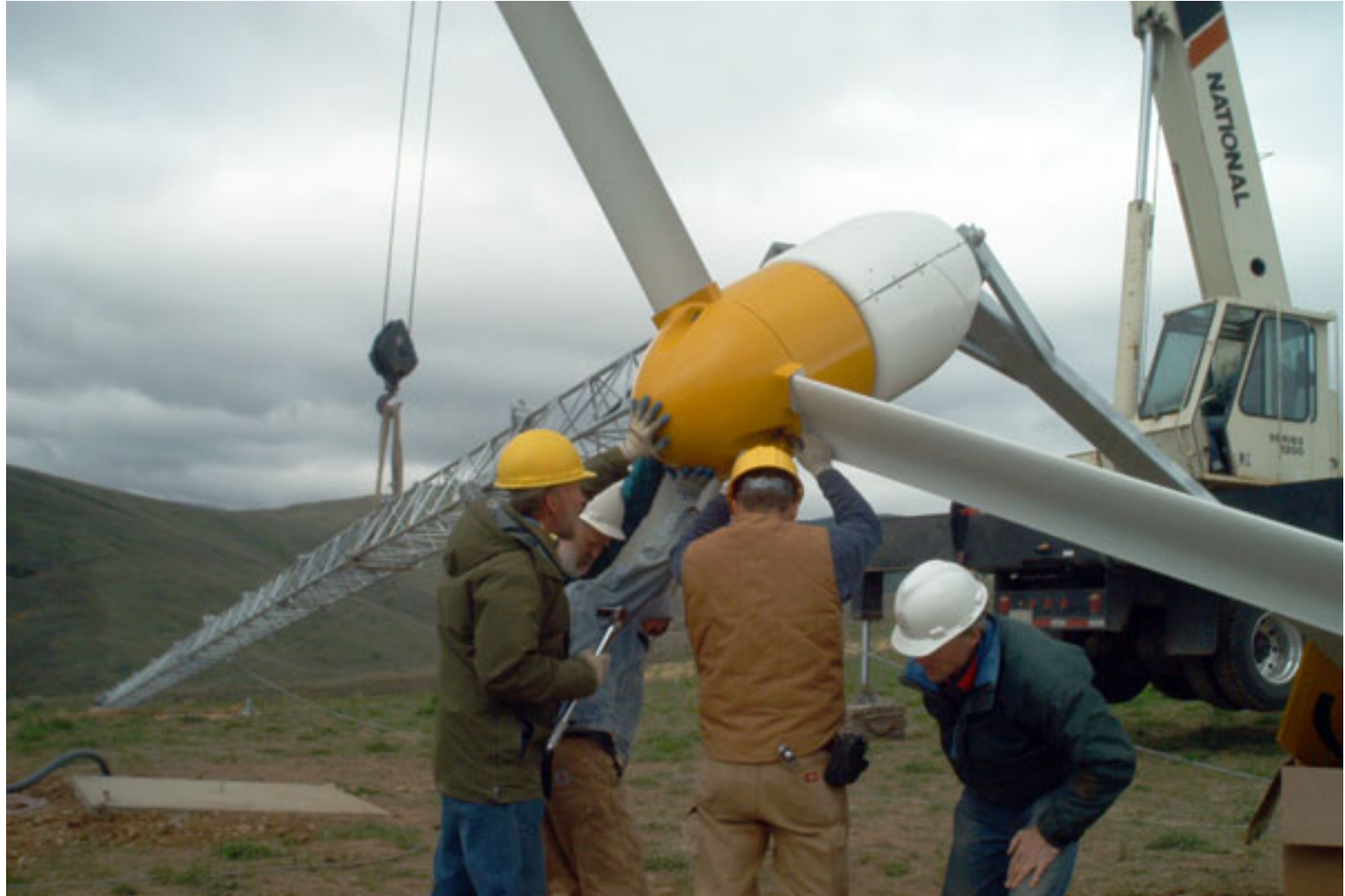
Wind turbine installation, courtesy DOE
