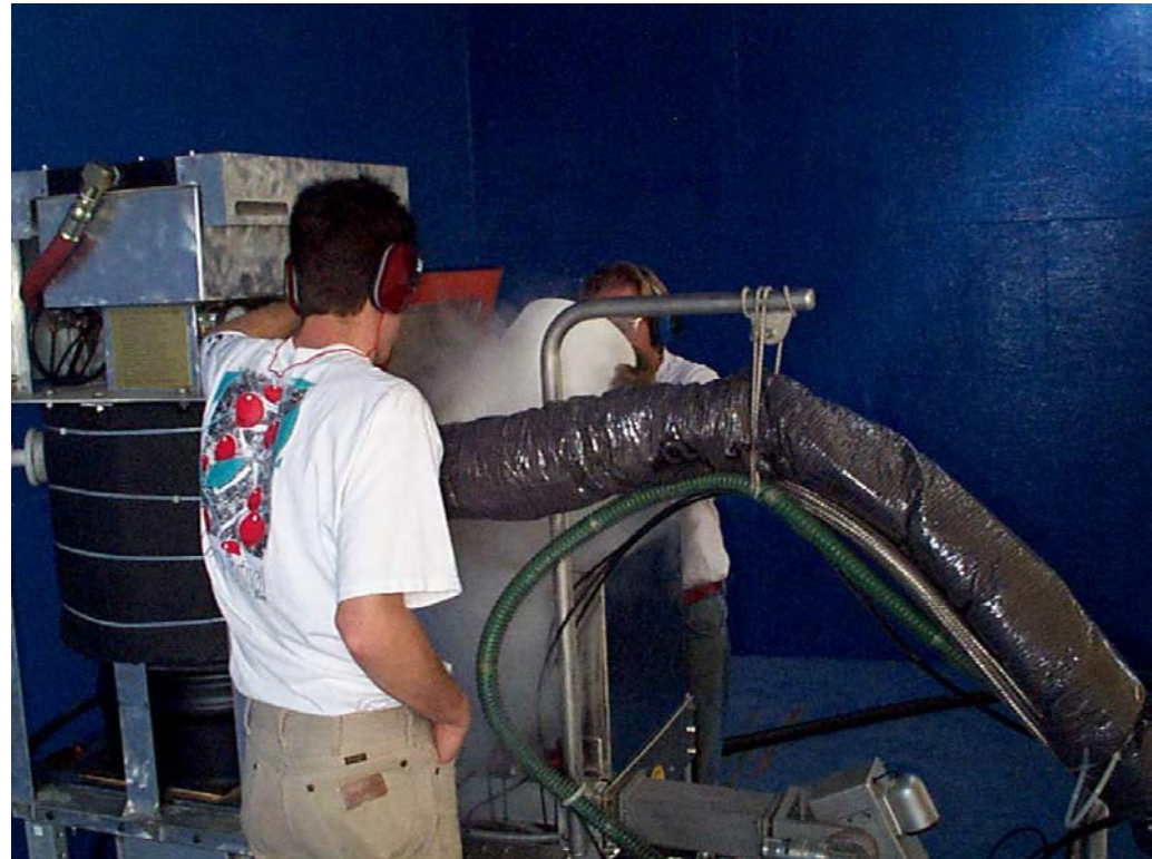
Dry ice blaster for radiation cleanup
