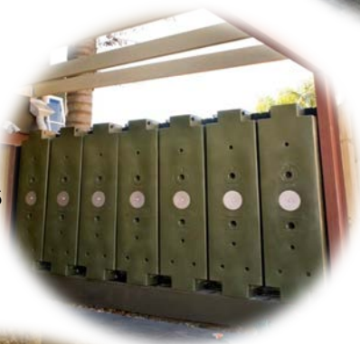
Rainwater catch basins
