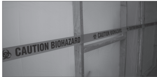
6-mil poly used as an engineering control.
