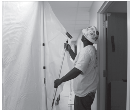
A plastic sheeting wall with an extension pole system
