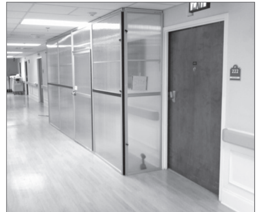
Modular wall-panel anteroom.
