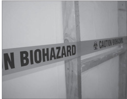
Decon built with 2"× 4" lumber and poly
