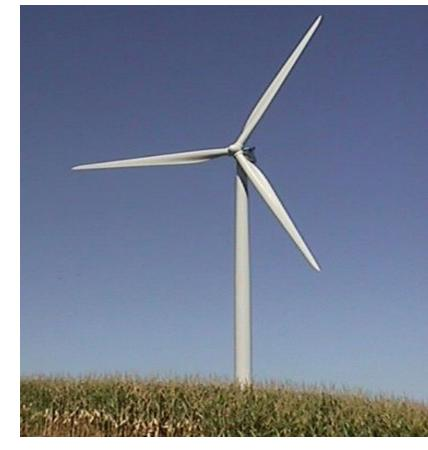
The wind turns the blades, which spin a shaft, which connects to a generator and makes electricity.
