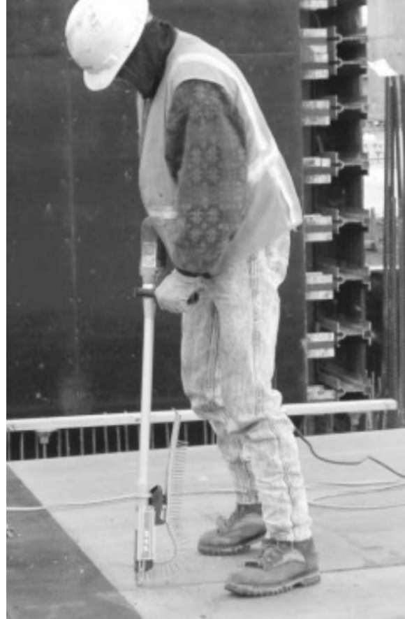
Solution: Autofeed stand-up screw gun
