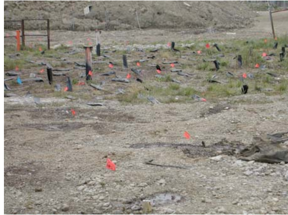
Figure 4: Flags Marking the Plugs Used Upon Completion of a Location.
