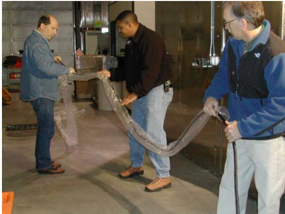
Figure 3: Workers Demonstrating Manual Sleeving of Cable.
