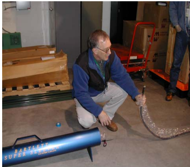
Figure 2: Engineer Demonstrating Sealing of Cable after Sleeving is completed.
