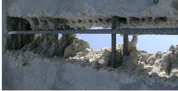
Figure 4: Close-up of Concrete after Hydrodemolition.
