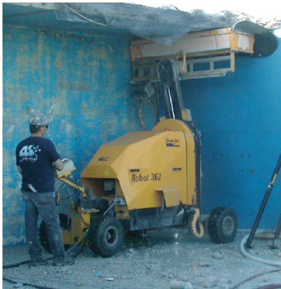
Figure 1: Operation of the Conjet Robot 363.
