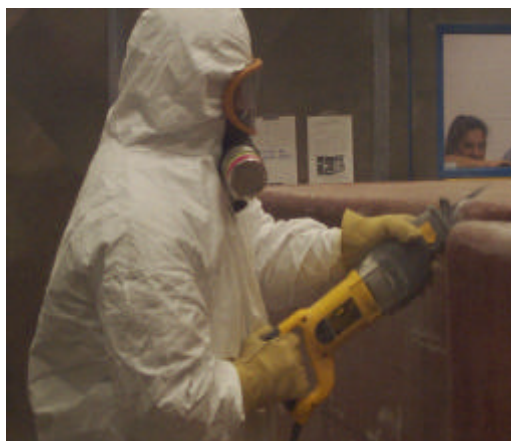
Figure 1. An operator beginning a cut in the vertical direction with the DeWalt Reciprocating Saw.
