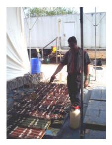
Electricity is routed from the rectifier (left) to bus bar (pictured on the left side of the right picture). Electrical leads are run from the bus bar and attached to the wire mesh inside the pads. The pads are held in place by magnets. Periodically the pads are sprayed with electrolyte to prevent overheating.
