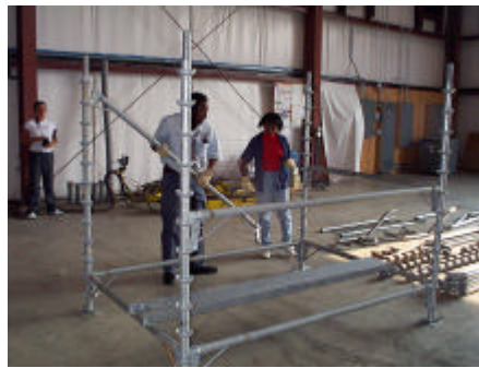
Users assembling the Excel Automatic Locking Scaffold System.
