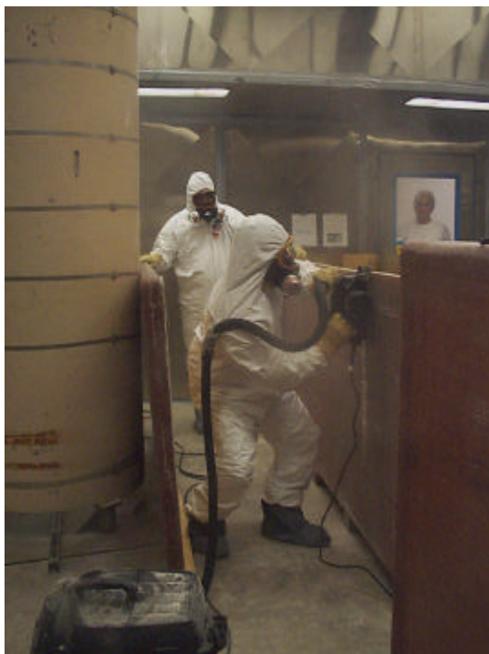
Figure 1. An operator making a vertical cut with the Porter-Cable Circular Saw. For this demonstration, the optional vacuum was attached to the directional nozzle.
