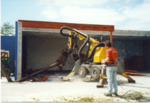
The La Bounty Shear is used to dismantle pipes.
