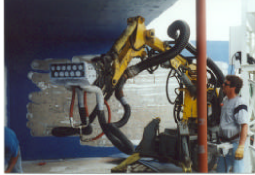
The articulating boom with SH-U11 scabbler attached.
