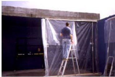
Figure 2. Containment being built around wall decontamination area.
